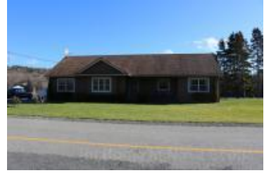
Contractor's home on the river
