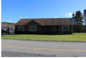
Contractor's home on the river
